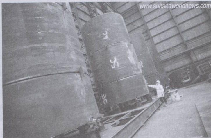
Under Construction of North Sea project
